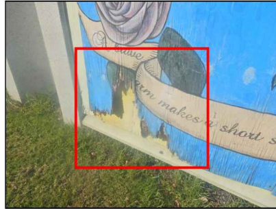
Damaged plywood
