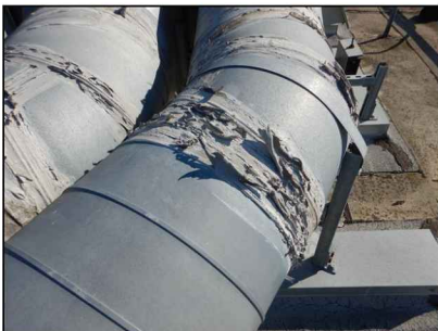
Deteriorated mastic
