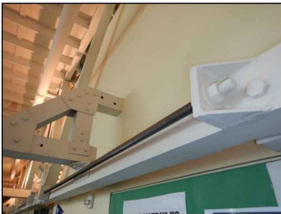
Truss modification
