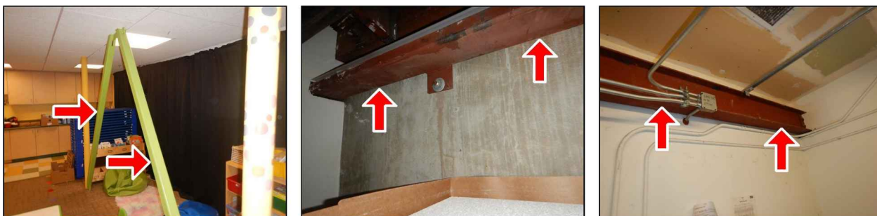
Seismic strengthening
