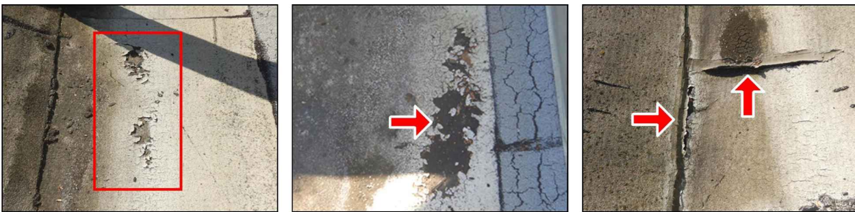
Worn roofing
