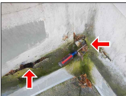
Rusted flashing
