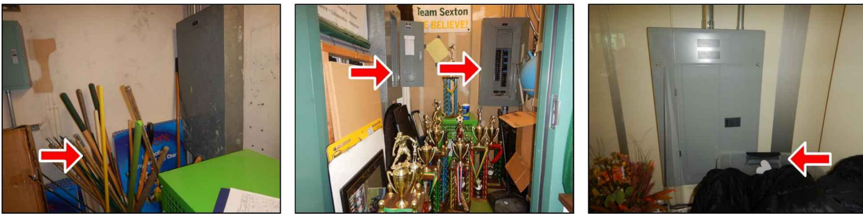
Blocked subpanels
