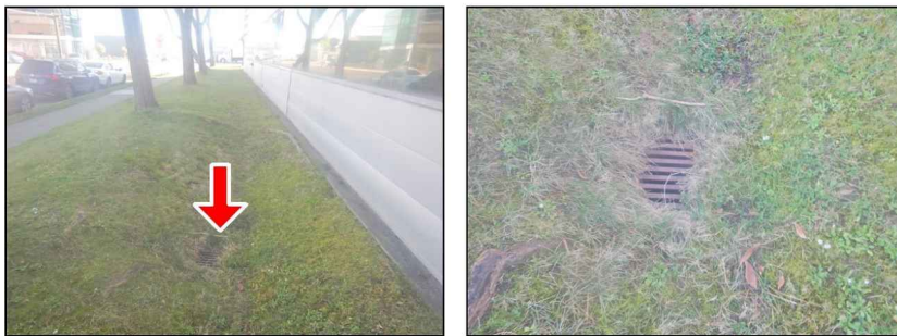
Perimeter surface drainage
