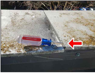
Open cap flashing joints
